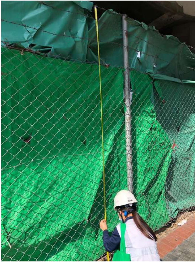
Figure A3 Hoarding along the site boundary
